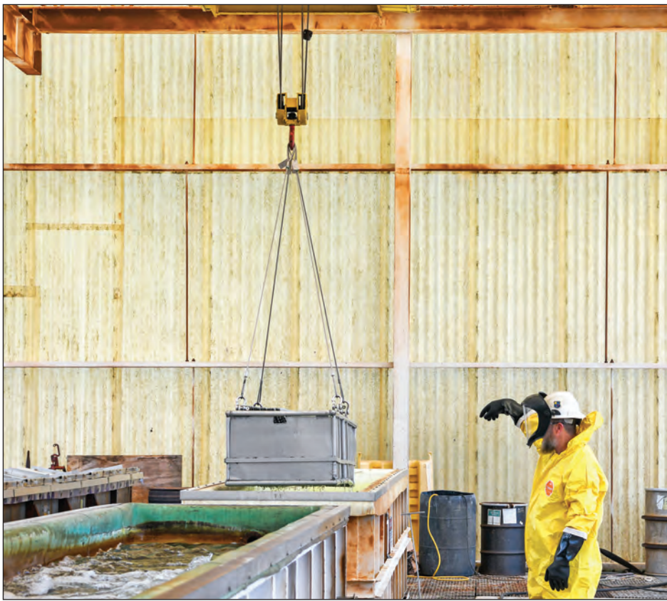
Scottie Stevens, an aerospace outside machinist, uses hand signals to direct a crane operator to lower a basket with an item to be cleaned June 29 in the chemical cleaning yard at Arnold Air Force Base. The vat contains one of two newly-acquired citrus-based cleaners purchased to replace hydrofluoric acid, a more dangerous chemical. Workers are able to wear less personal protective equipment with the new cleaner. Stevens is wearing a Tyvek suit, but had he been wearing long sleeves, he could have worn an apron instead, in addition to the gloves and face shield. (U.S. Air Force photo by Jill Pickett)
