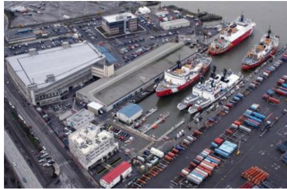
Aerial View (from the North) of Base Seattle.
