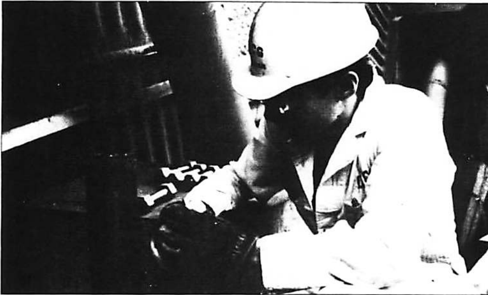
Marine Inspector inspects boiler safety valve mounting bolts.
