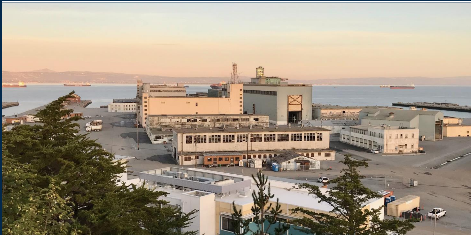
View of Parcel C at Hunters Point Naval Shipyard
