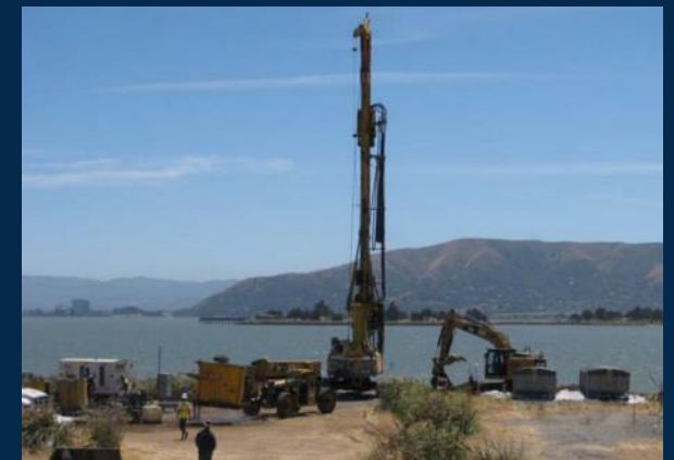
In situ stabilization of oily waste at Parcel E
