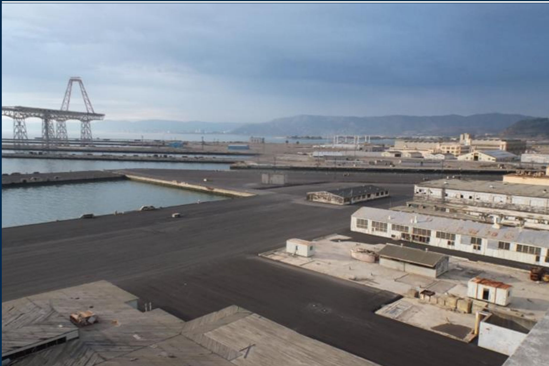
Durable covers of asphalt and buildings are part of the final remedy at Parcel C Aerial view of Parcel C, looking towards the gantry crane on Parcel D-1
