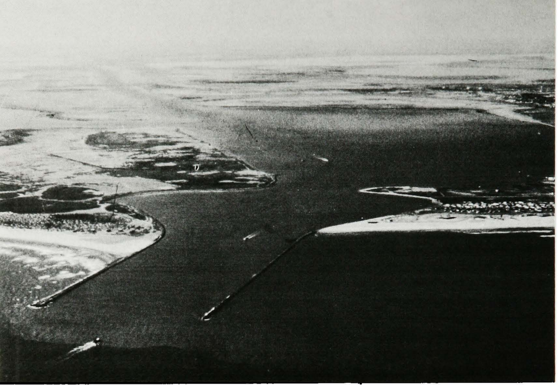
Completed jetties at Brazos Santiago. Brownsville Ship Channel veers to the left in background.
