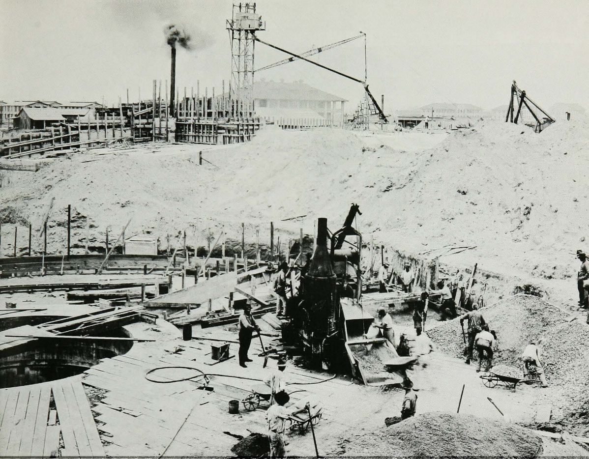
Construction of gun well for 12-inch battery at Fort Crockett, 1918
