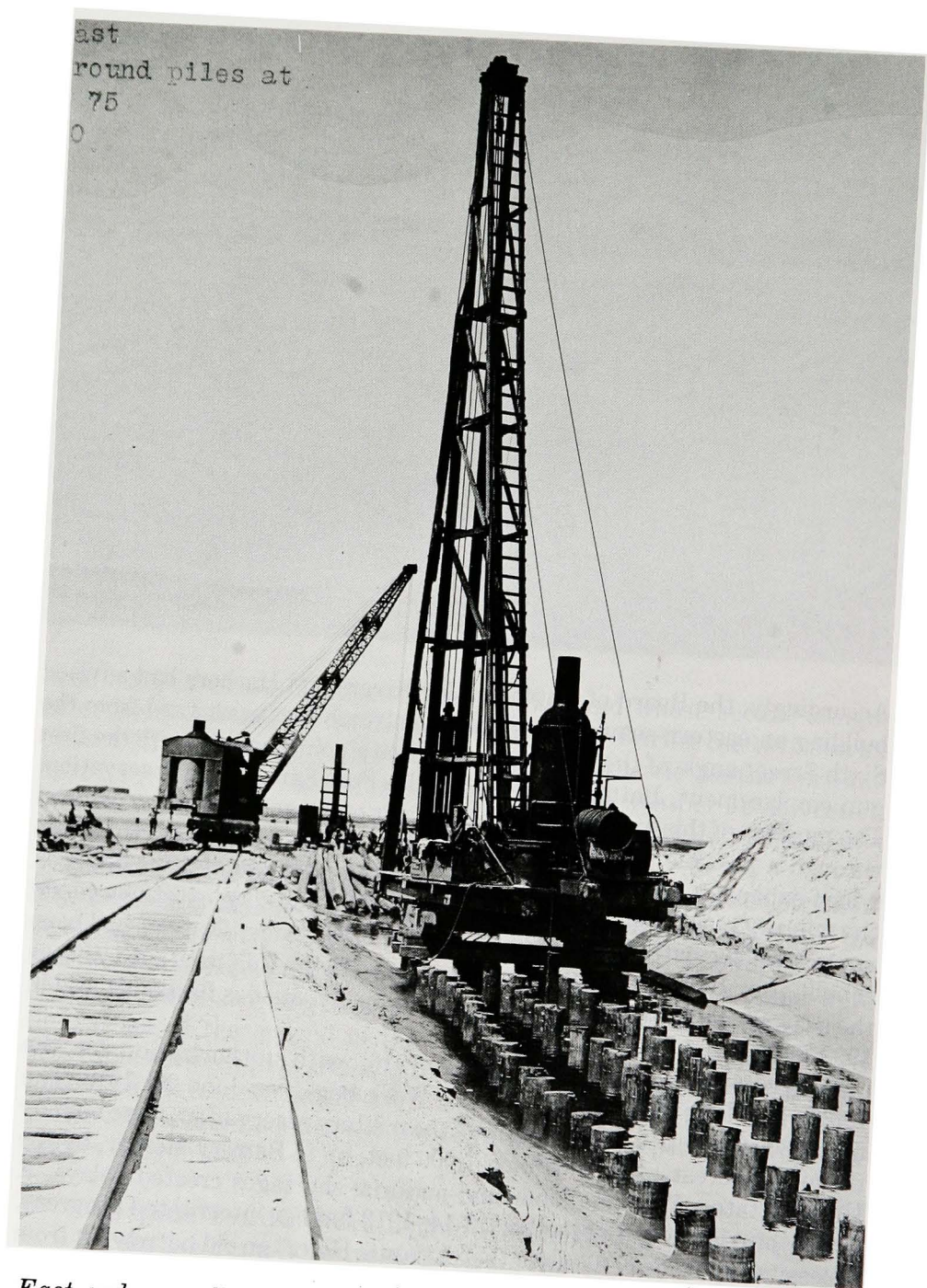
East end seawall extension. Pile driver placing round wooden piles, May 17, 1920
