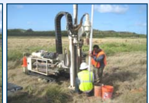
SWMU 56 – GeoEnviroTech drillers installing a groundwater monitoring well
