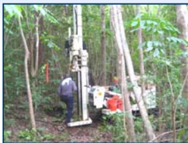
SWMU 62 – JFA Drillers collecting subsurface soil samples
