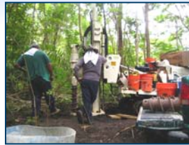
SWMU 61 – JFA Drillers installing a groundwater monitoring well
