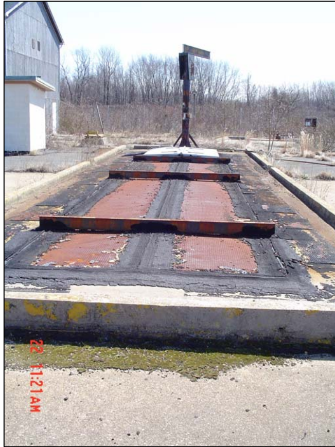
Photo 3: Cover of former underground Nike missile magazine elevator.
