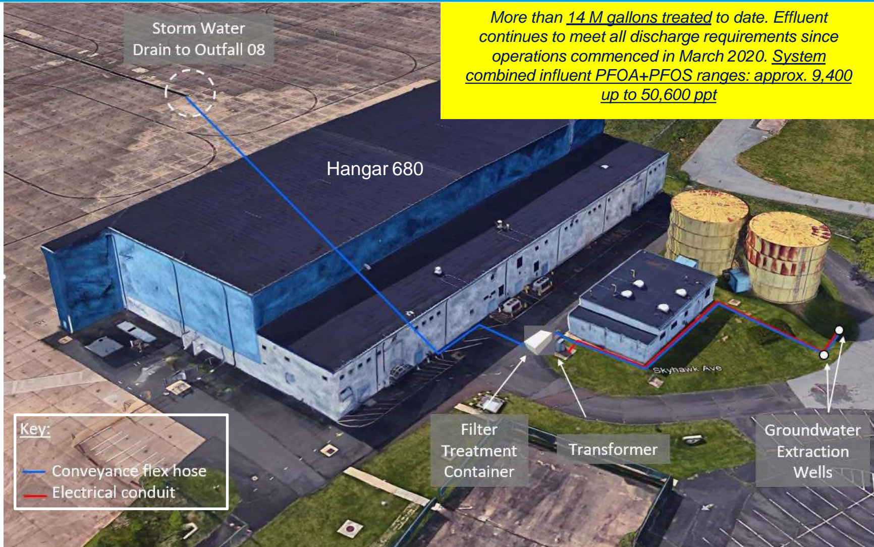
Location of Hangar 680 treatment system
