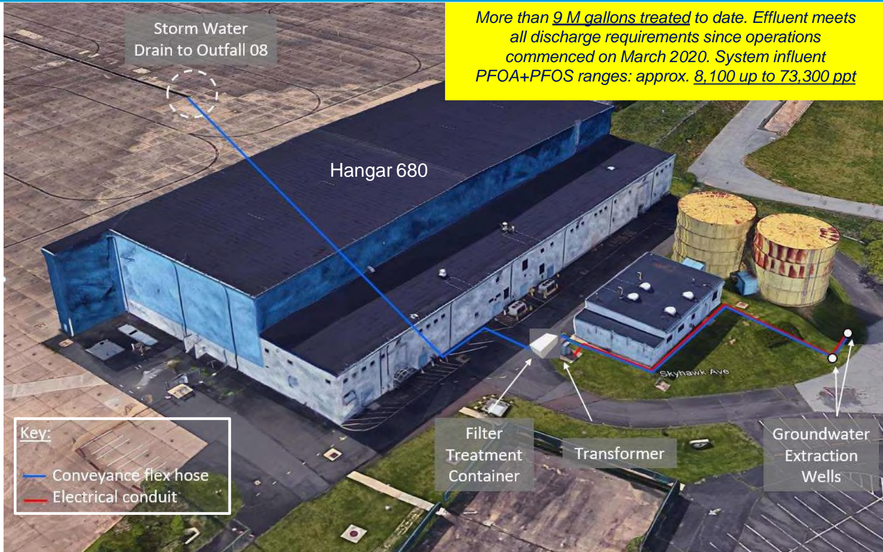
Location of Hangar 680 treatment system
