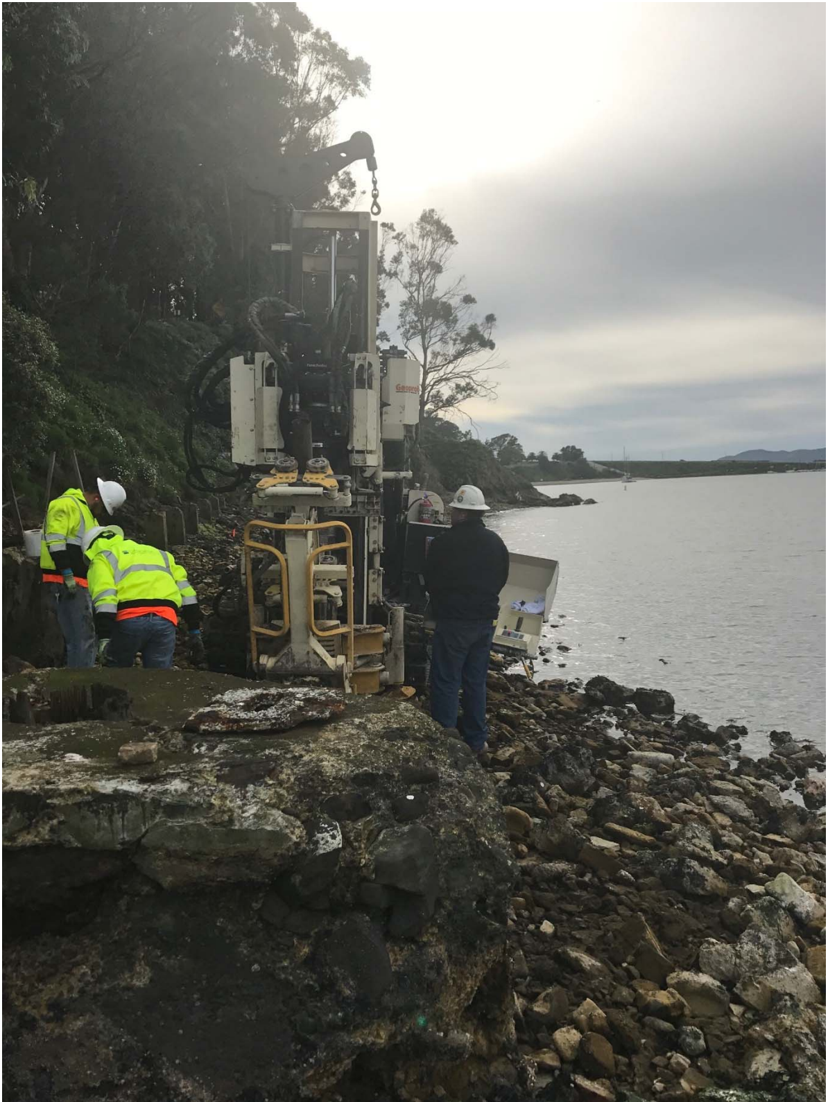
Photograph 3. Collecting sediment core with Sonic drill rig at location YF307.
