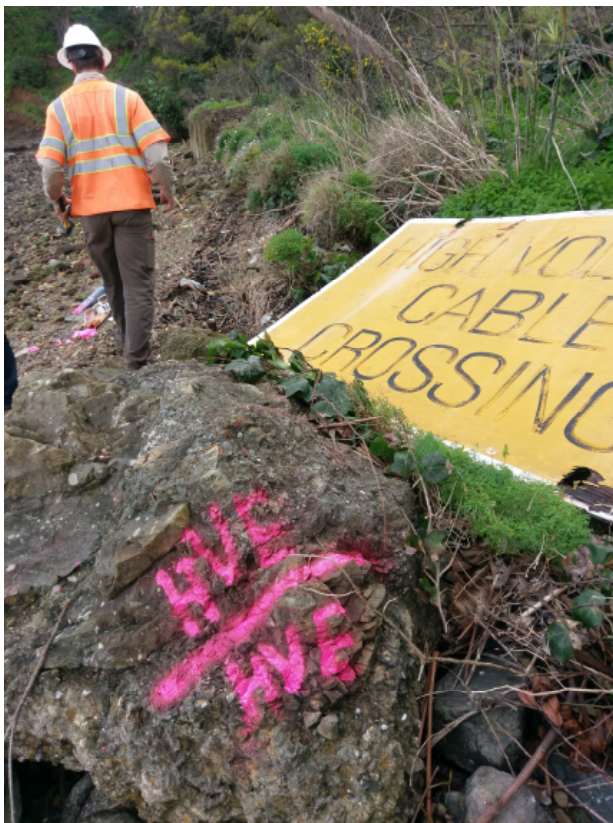
Photograph 2. Utility marking of high voltage line on rock at Site YF3.
