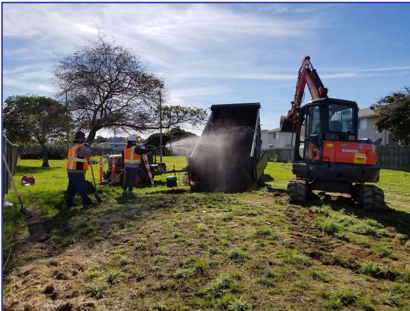
Dust Control Measures at Site 12 Excavation Area
