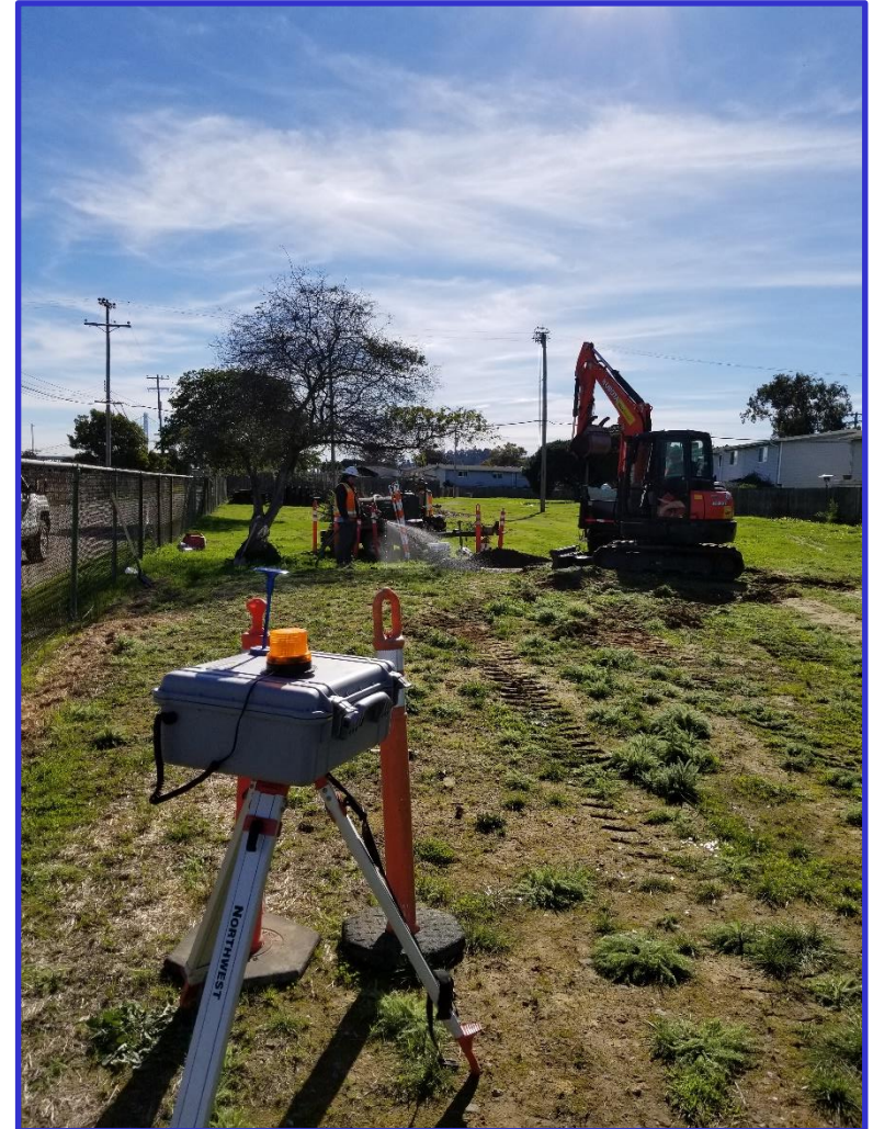
Dust Monitoring at Excavation Location
