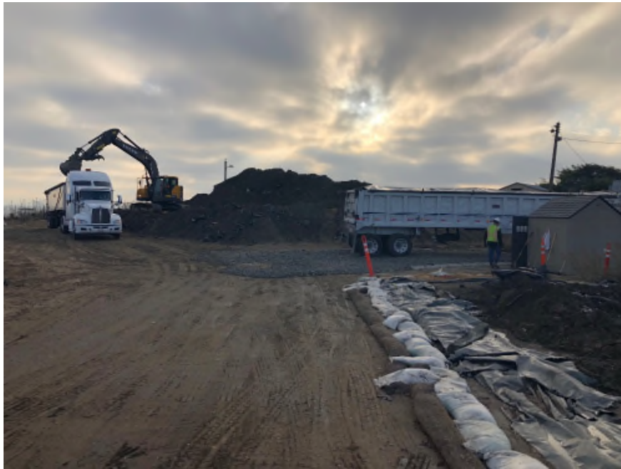
Loading Soil Stockpiled at Site 32 for Off-Site Disposal: Buttonwillow, CA Landfill
