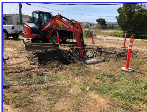
Halyburton Court excavation
