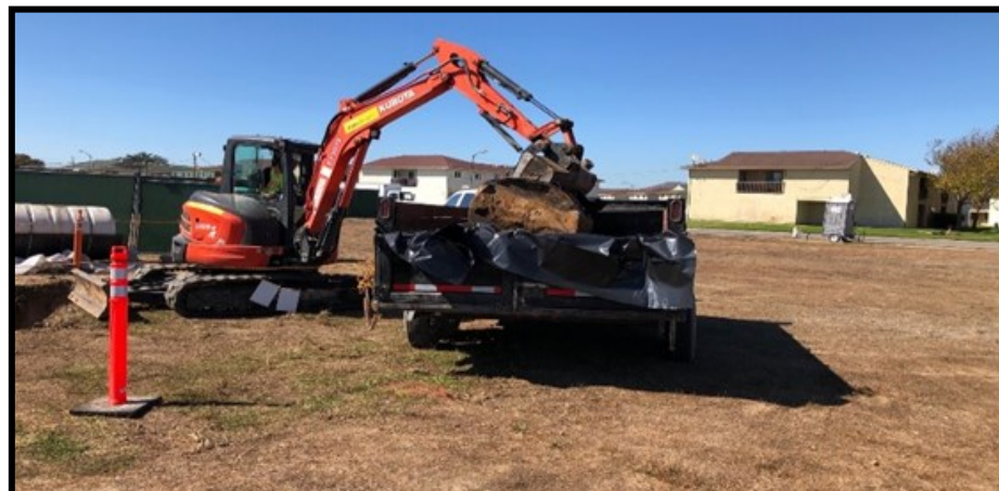
Photograph 6: Removal of underground storage tank
