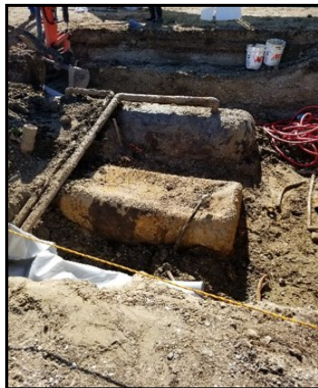
Photograph 8: Underground storage tanks
