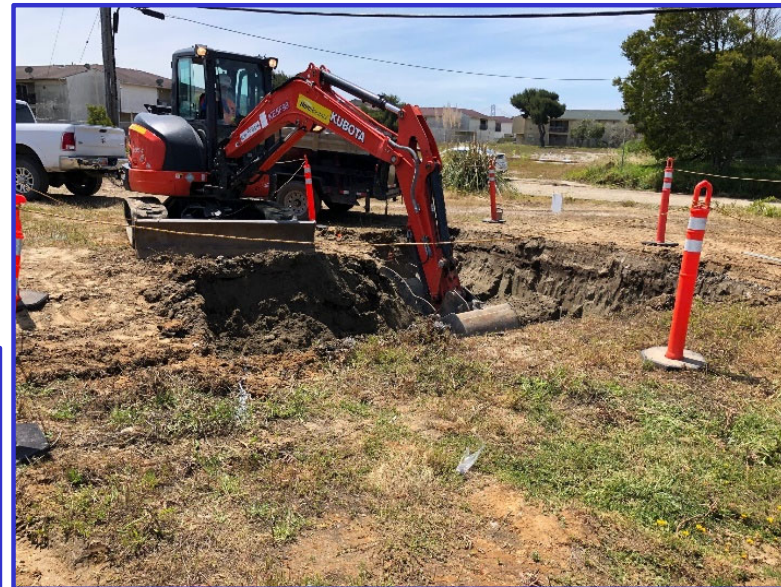
Example of discrete excavation. Excavation and Backfill at Haliburton Court.
