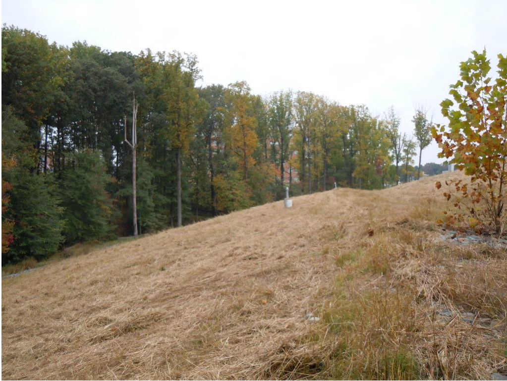
OU2/OU3 - Southern Slope of Landfill with Gas Vent
