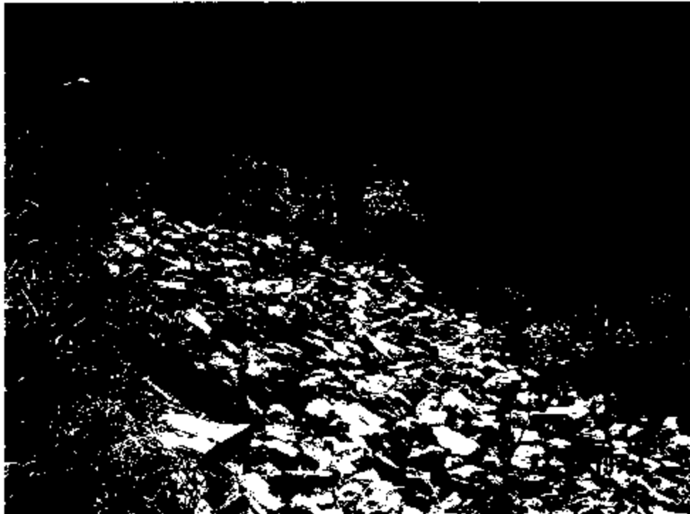
OU2 Landfill, Photo 7 – Rip-rap for stabilization along toe of landfill, looking east.
