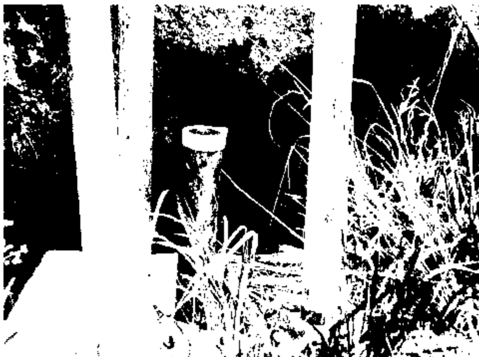
OU2 Landfill, Photo 11 – Monitoring well next to unnamed tributary, missing cover.
