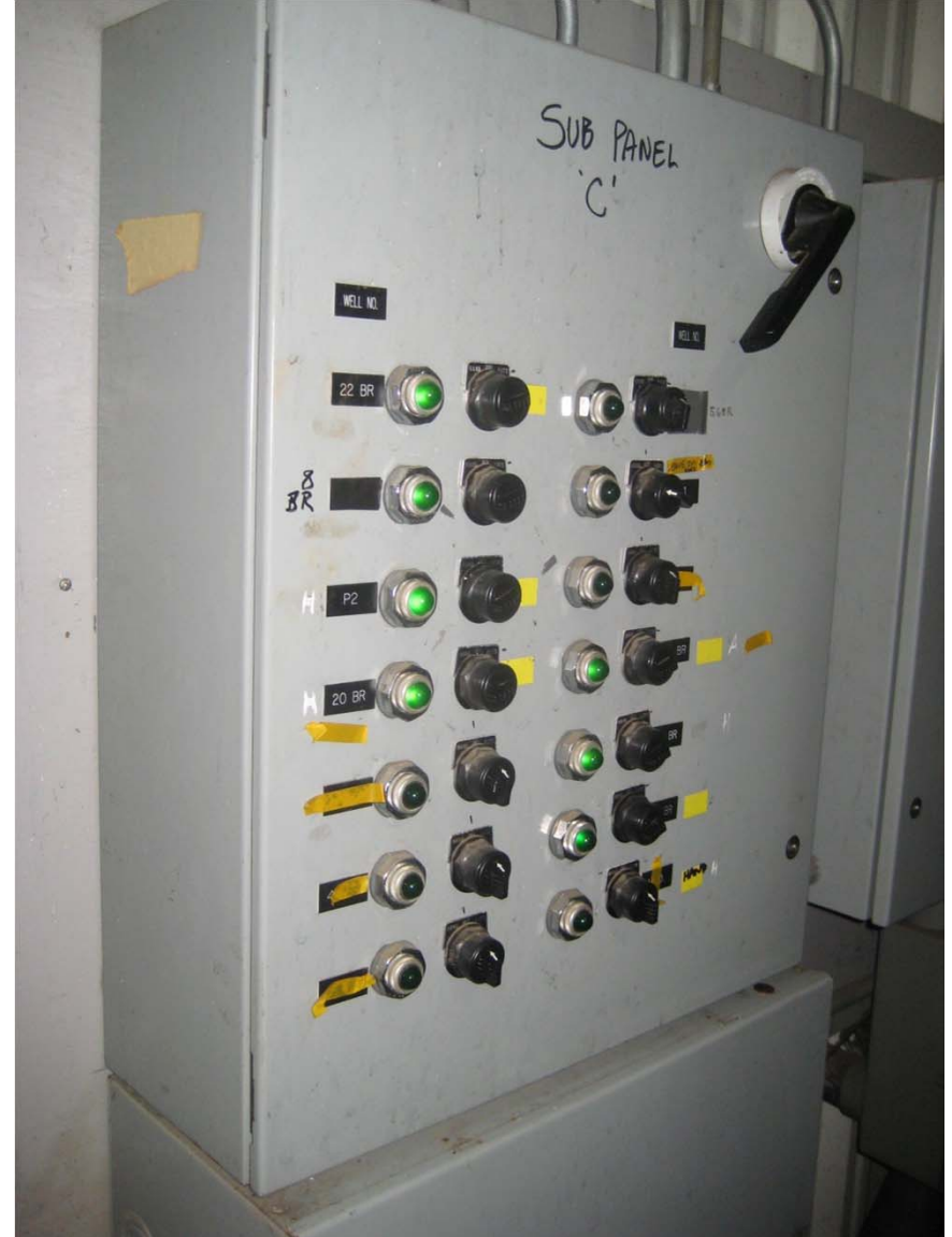
Extraction Well Control Panel
