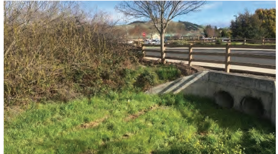
Photo 8: Dense willow growth appears to be providing flow obstruction within the main channel upstream of Silver Oak Trail. The culverts shown in the foreground provide overflow capacity (March 2018).
