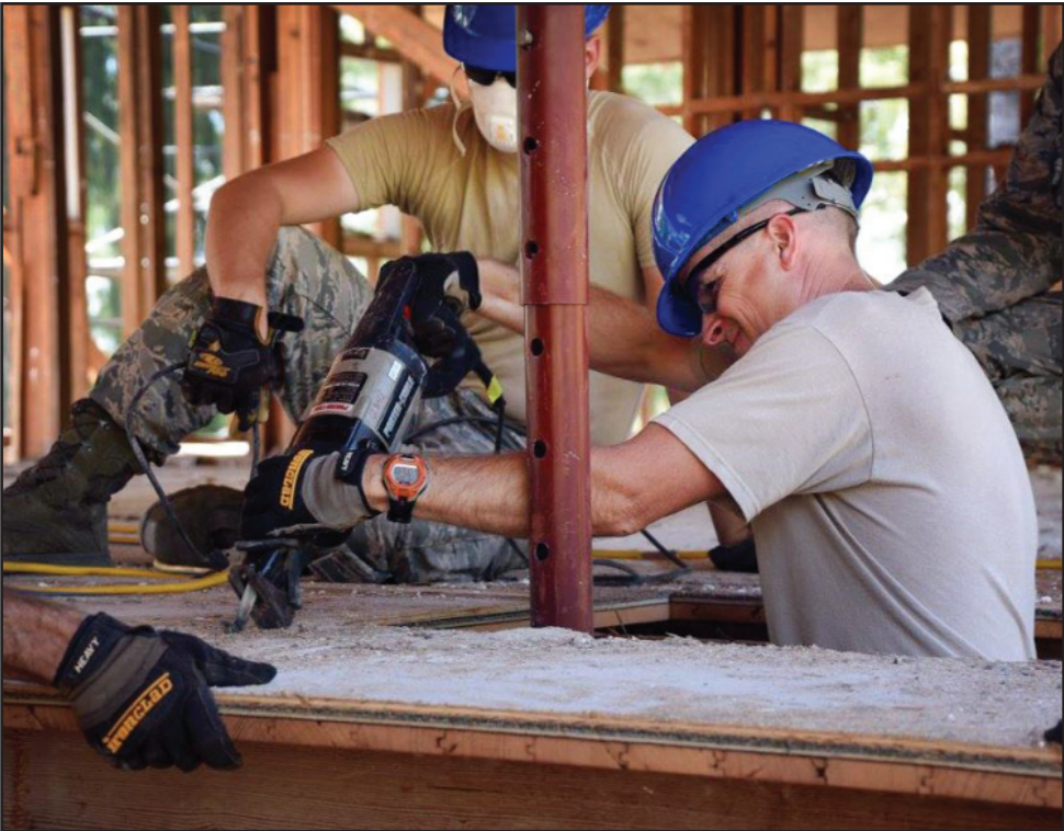
Engineers with the 184th Civil Engineer Squadron use a reciprocating saw to make a cut during a construction project at Bellows Air Force Station, Hawaii. (Photo by Staff Sgt. Lauren Penney, 184th Intelligence Wing Public Affairs)
