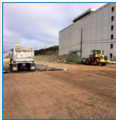
Truck beds containing soil are required to be covered
