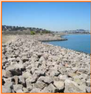
Rock walls minimize dust along the shoreline
