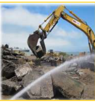
Water is used to minimize dust at active construction sites
