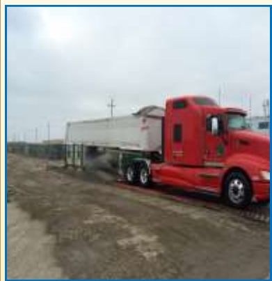
Before exiting HPNS, trucks pass through the tire wash and over rumble strips
