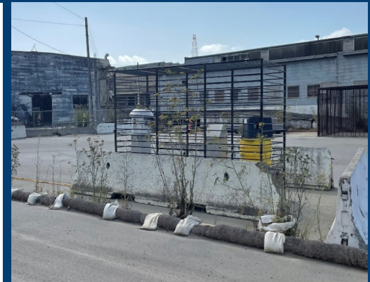
Air monitoring stations are placed upwind and downwind of active construction areas
