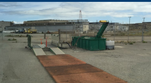
Rumble strips shake excess dust from truck tires
