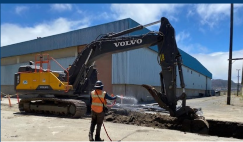
Workers use water to reduce dust during construction
