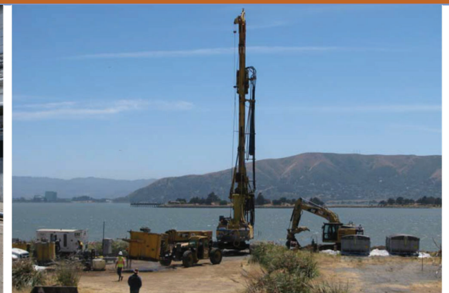
In-situ stabilization of oily waste at Parcel E
