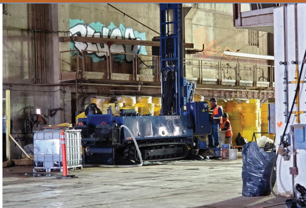
Eco-friendly groundwater treatment at Parcel C
