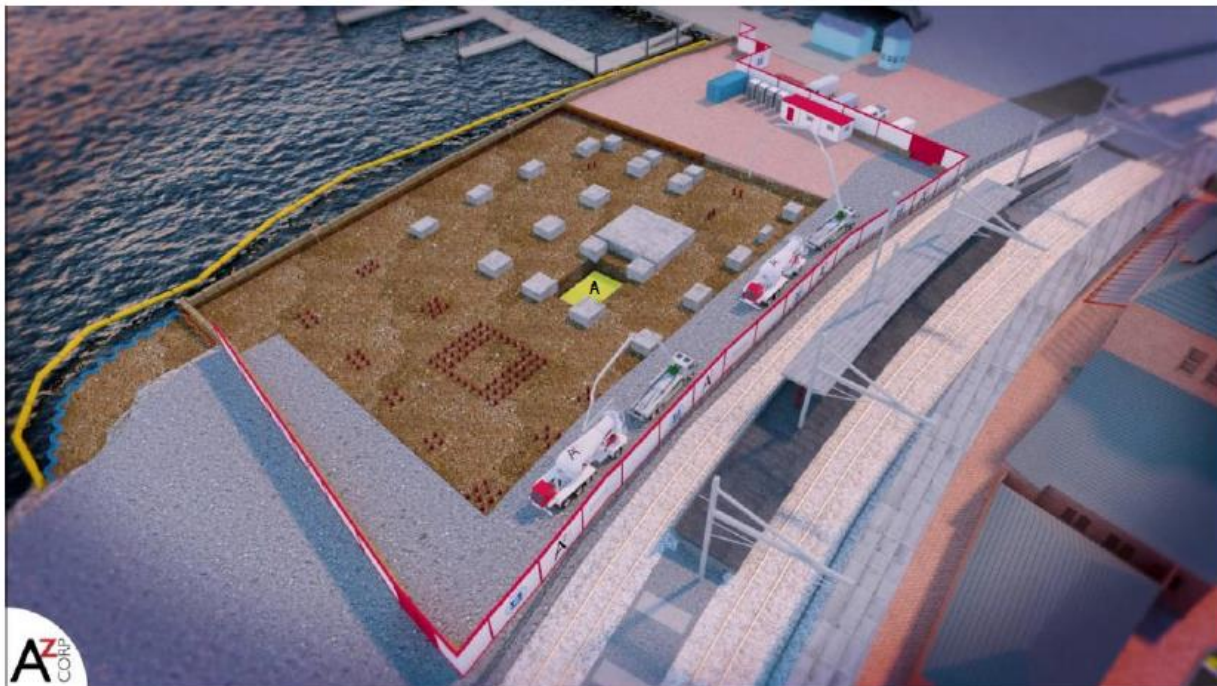
Figure 2.3-16: Pile Driving Operations and Pile Cap Construction
