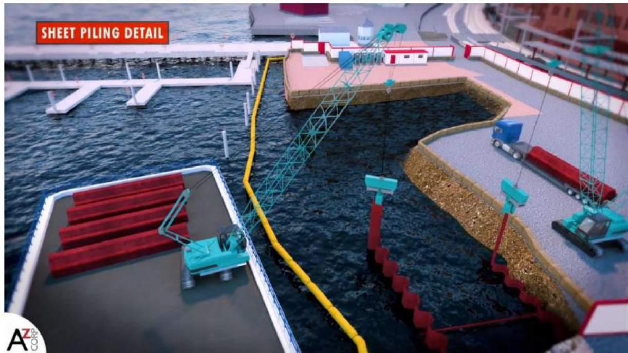
Figure 2.3-14: Barge and Pile Driving
