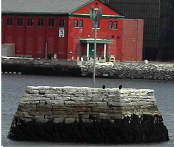
Photo 5-1 - Stone Foundation Aid
