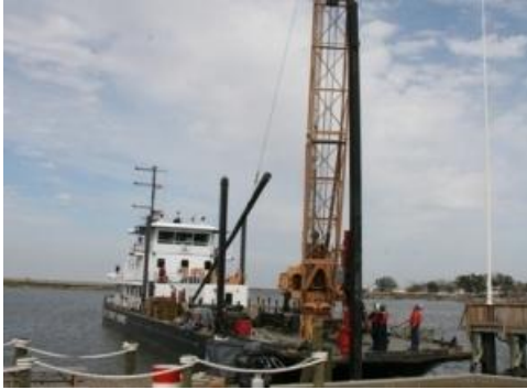
Figure 12-5 Crane Hoisting Pile
