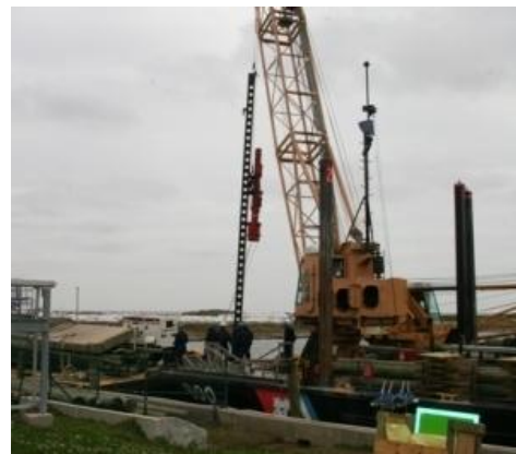
Figure 12-4 Hoisting Hammer and Lead
