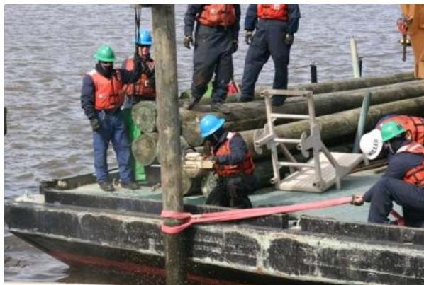
12-7 Cutting Pile Top
