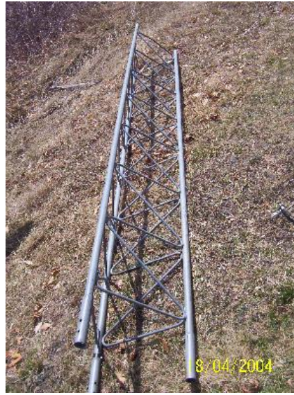
Figure 11-11 10ft Rohn Tower Section
