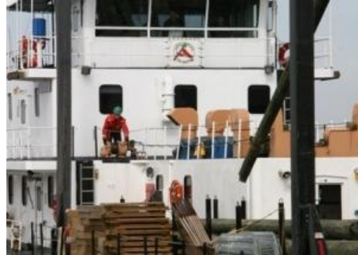
Figure 12-6 Cross Deck Winch Easing Out Pile
