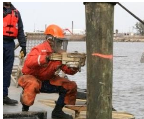
12-8 Cutting Pile Top
