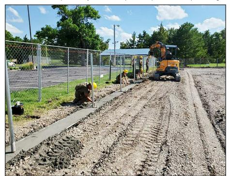
Members of 226th Engineer Company finish a section of a concrete mow strip and prepare another prior to installing a new fence at the Hays armory bullpen during annual training July 11-25.
