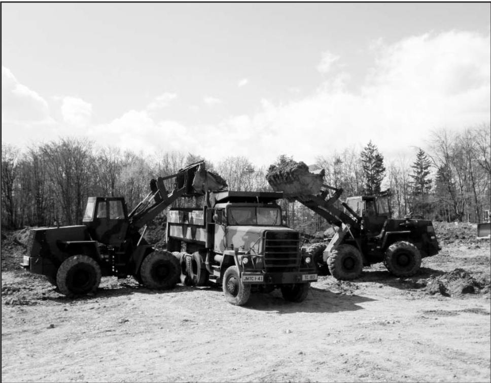
Staff Sgt. Jared Ludwig and Sgt. Timothy Shoulders, 242nd Engineer Company, Kansas National Guard, load a 20-ton dump truck with fill dirt for the CH47 pad expansion project in Hohenfels, Germany. (Photo by Spc. Maureen McWilliams, UPAR, 242nd Engineer Company)
