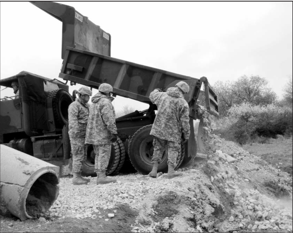
Staff Sgt. John Lyon directs Sgt. Vernon Valentine where to dump rock as Sgt. Donald Vining and Spc. Daniel Fogle observe. The rock will be compacted to allow for a stable base for a culvert at the IED Lane north project area in Hohenfels, Germany. (Photo by Spc. Maureen McWilliams, UPAR, 242nd Engineer Company)
