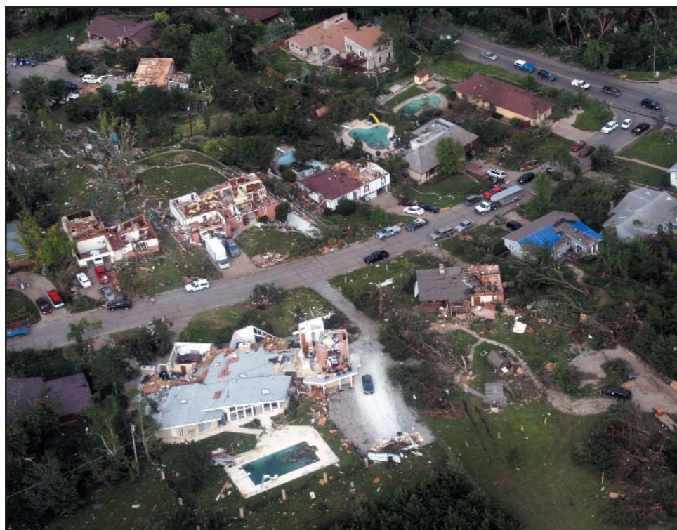
An EF4 tornado skipped through Manhattan, Kan., the evening of June 11, striking business and residential areas alike. The Kansas State University campus sustained an estimated $27 million in damages. (Photo by Sharon Watson)
