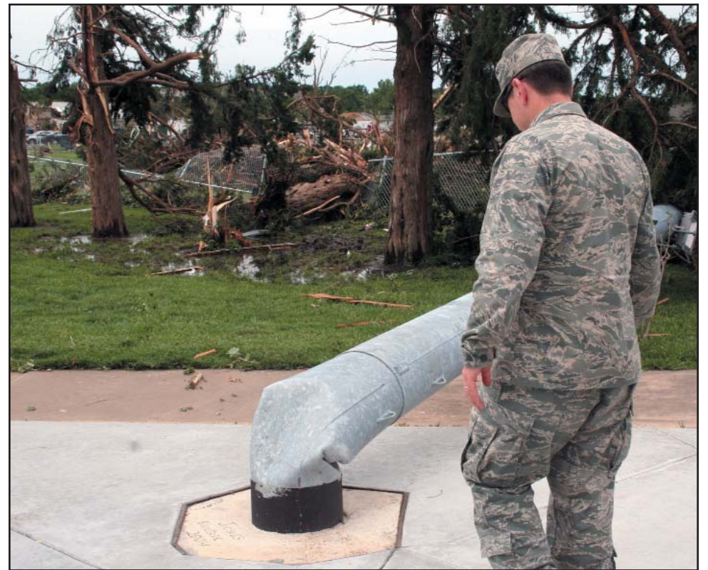
Maj. Gen. Tod Bunting, the adjutant general, examines a light pole at the high school football field, bent by the force of the tornado. (Photo by Sharon Watson)
