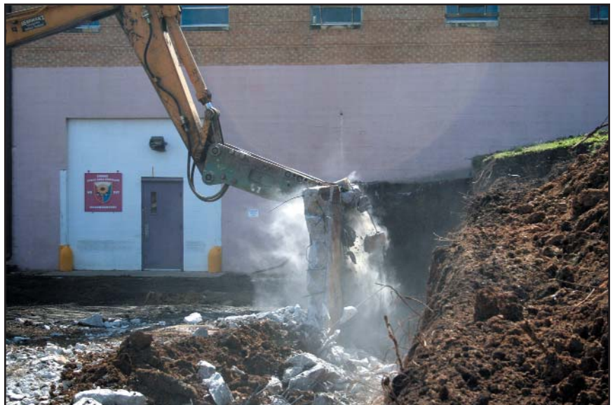
Construction workers use a crane operated jack-hammer to demolish a retaining wall in preparation for renovations at Nickell Armory in Topeka.
