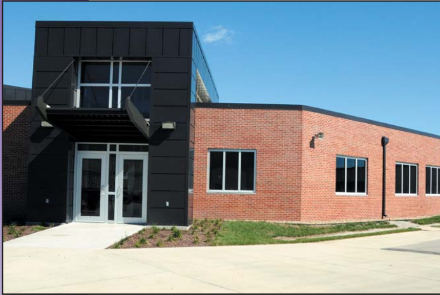
190th Civil Engineers moved back into their newly renovated 14,690 square-foot facility.
