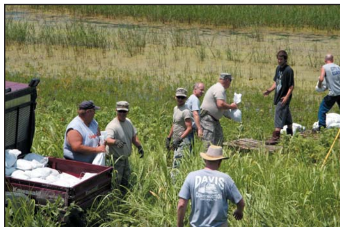
Soldiers of the 2nd Battalion, 130th Field Artillery assist with repair of a sand boil along a levee near Elwood, Kan. The soldiers were deployed to Doniphan County to assist local authorities with flood control measures.
