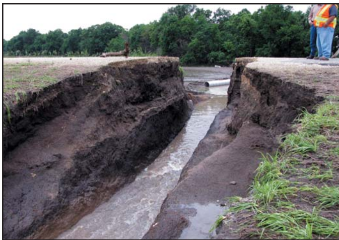
Floodwaters washed out these drainage tubes on Highway 24 near the Missouri River.
