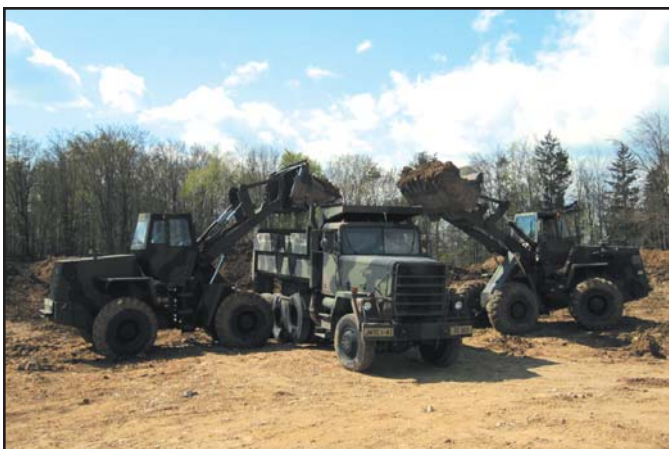
Soldiers of the 242nd Engineer Company load a 20-ton dump truck driven by a 242nd soldier with fill for a helicopter pad expansion project in Hohenfels, Germany.
