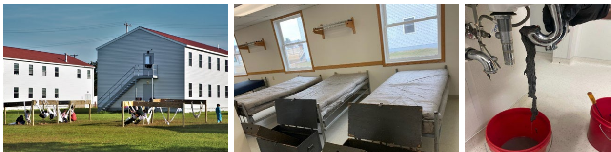
Figure 3. Fort McCoy Barracks used during OAW and a clogged pipe Source: Fort McCoy.
