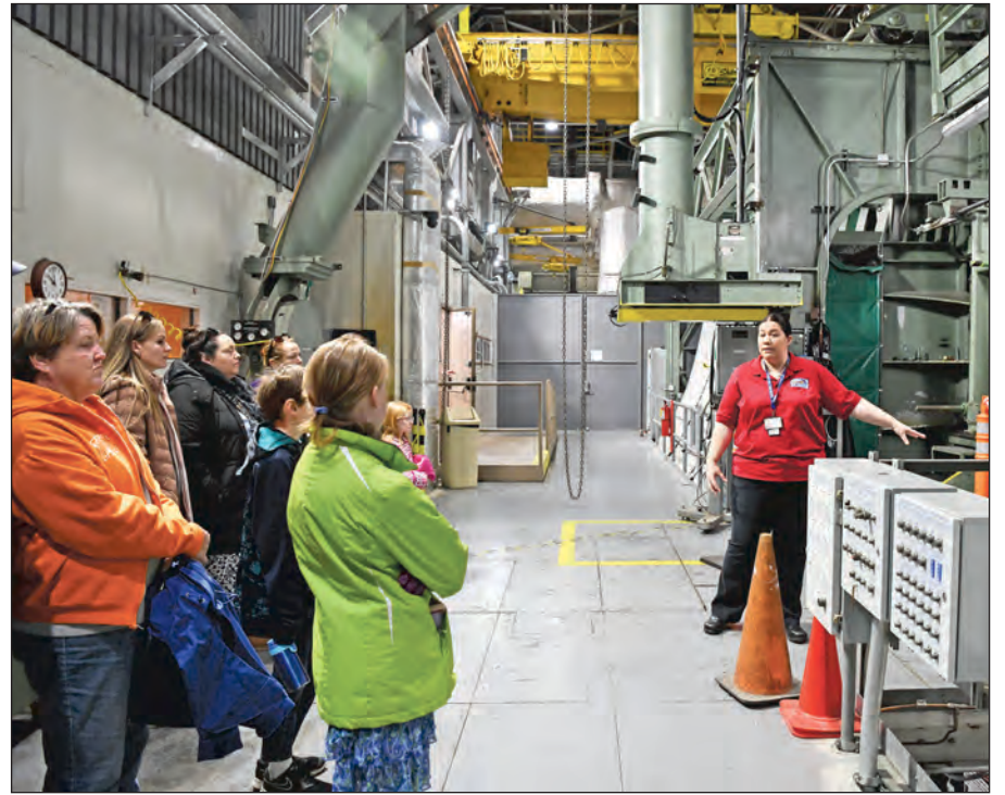
Arnold Engineering Development Complex team member Rebecca Rought speaks about Tunnel A in the von Kármán Gas Dynamics Facility to attendees of the 716th Test Squadron Open House and Family Day Nov. 21 at Arnold Air Force Base. (U.S. Air Force photo by Jill Pickett) (This image has been altered by obscuring one or more badges for security purposes.)
