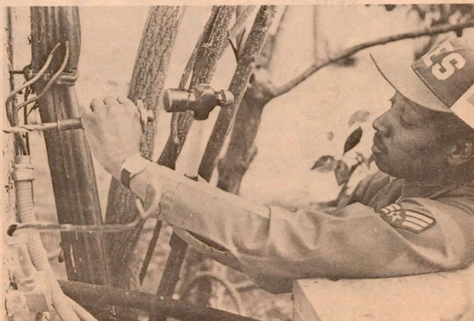
Sgt. Donald Gambrell, an internal electrician, taps a hole in the wall of a house for installation of a junction box.
