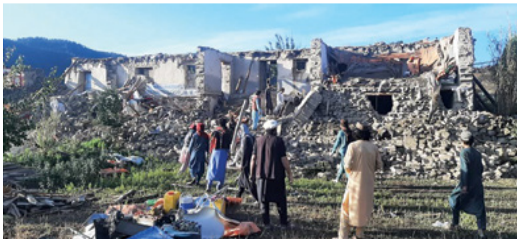
Destruction from the June 22 earthquake in southeastern Afghanistan. (WFP photos)
