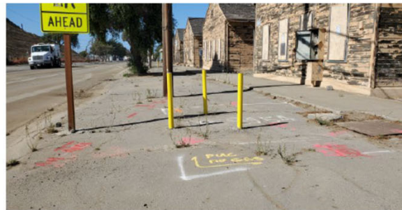
Typical bollard installation, embedded about 2' and filled with cement
