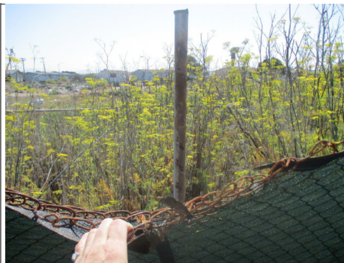
SWDA Westside Site 12: View of fence post detached from fence mesh. View to E.
