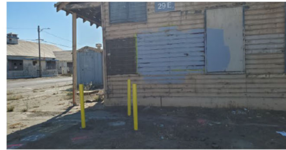
Typical bollard installation, embedded about 2' and filled with cement
