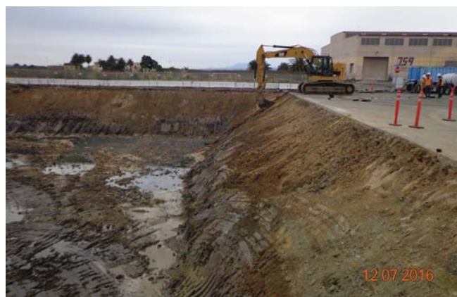
Chlorinated solvent area soil excavation at the IR17 and Building 503 Area
