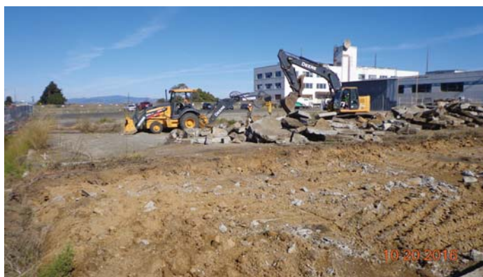
Concrete removal at IR17 and Building 503 Area prior to excavation
