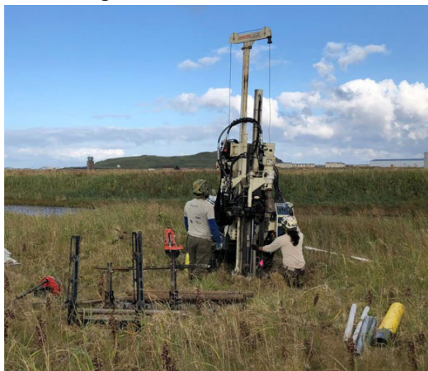
Monitoring Well Installation
