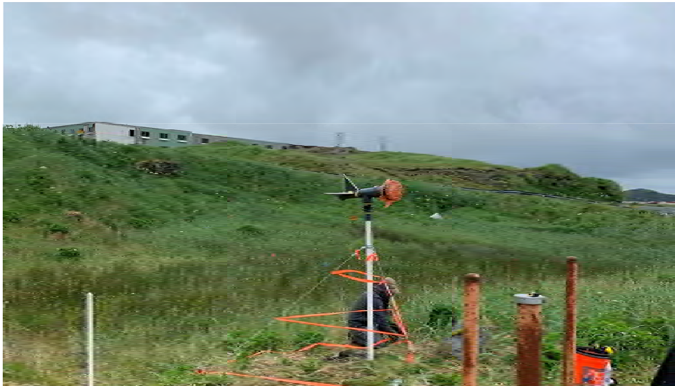
Installed Biovent Well and Vapor Monitoring Points
