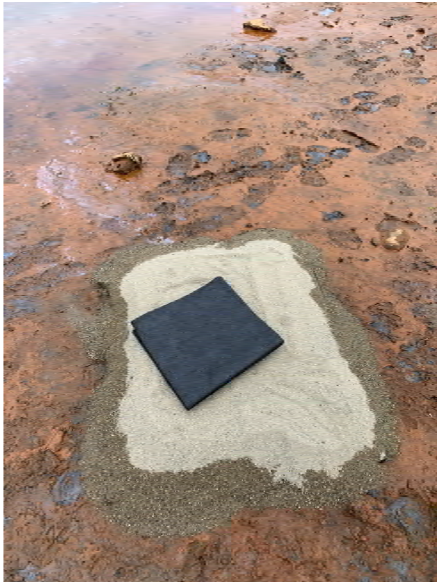
OBB prior to geotextile and anchor rock placement
