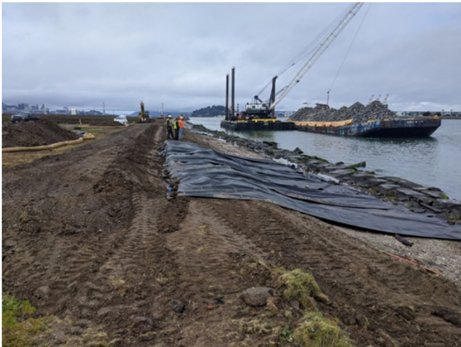
Shoreline Stabilization operations at Site 1. Crane barge and materials being barged and staged in Oakland Inner Harbor, also showing stabilization work next to training wall.
