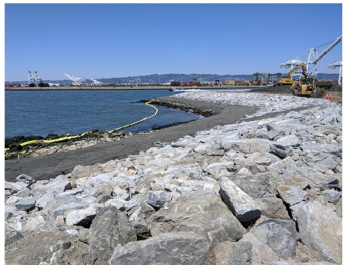
Northwest corner of IR Site 1 with beach berm installed.
