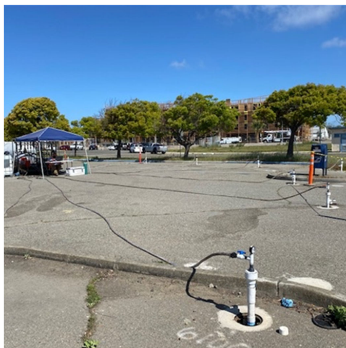
Injection Wells at OU 2B during the April to May 2020 injection event.
