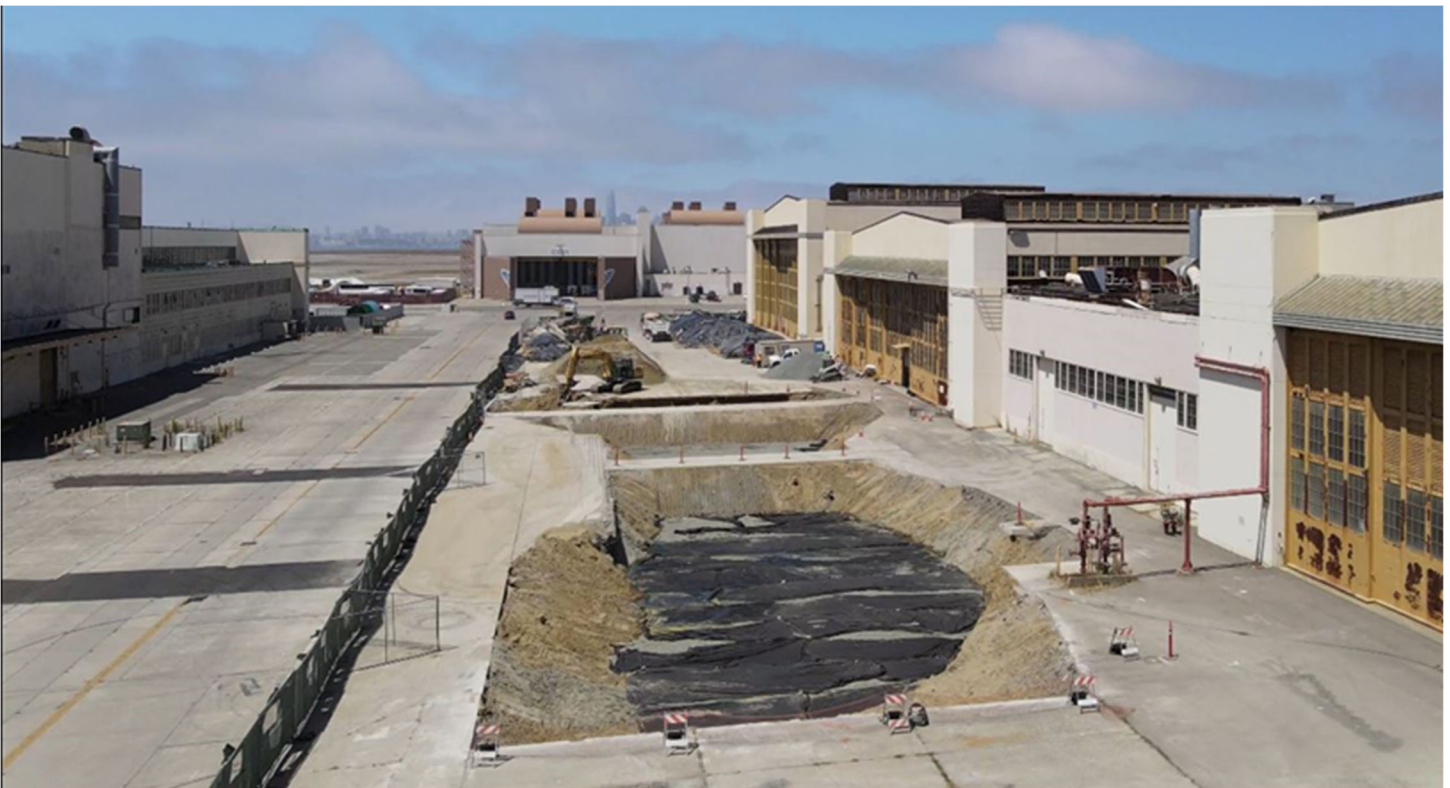
Excavation at Corrective Action Area 5B West to remove petroleum-impacted soil. Source: Richard Bangert
