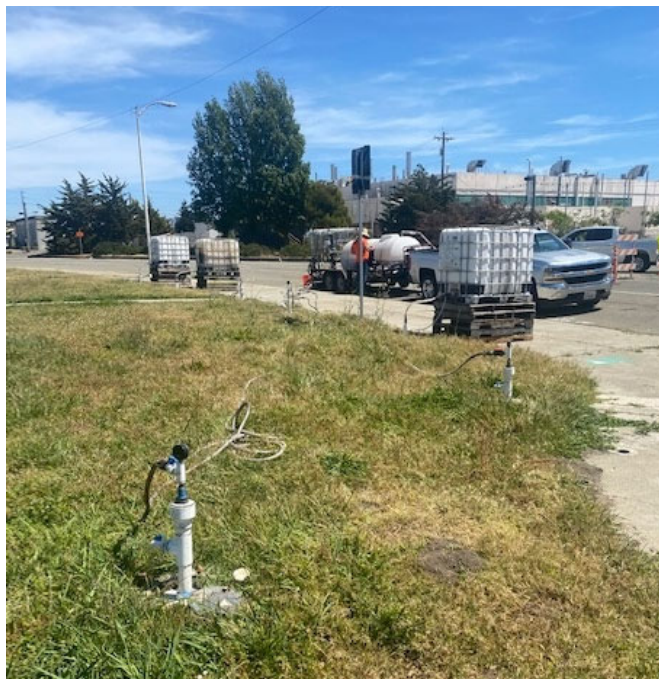
Injection Wells at OU 2B during the April to May 2020 injection event.
