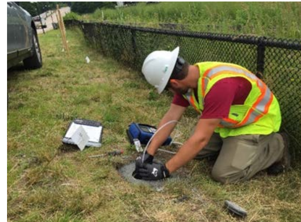
Photo of methane monitoring at temporary gas probes north of RDA
