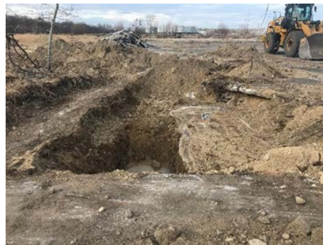
Photo of test pitting activities in the southern hangar slab area
