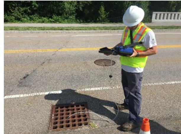
Photo of methane monitoring at utility access points
