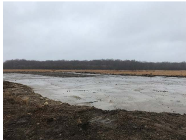
Photo of cleared northern hangar slab area
