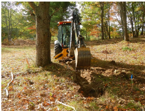
Test Trenching
