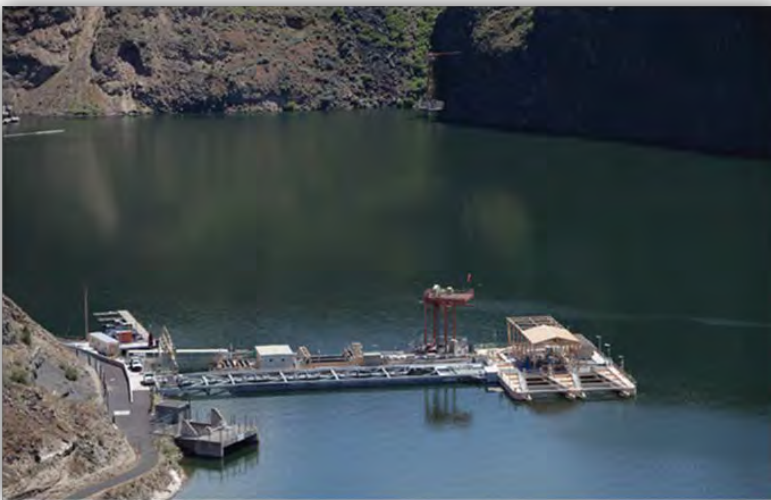
Figure 3-11. Floating Surface Collector (Lake Billy Chinook, OR)
