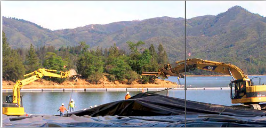
Figure 3-3. Whiskeytown Submerged Weir Installation
