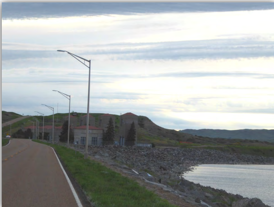
Figure 3-8. Intake Gate Houses at Fort Peck, Showing both Ring Gate and Roller Gate Houses
