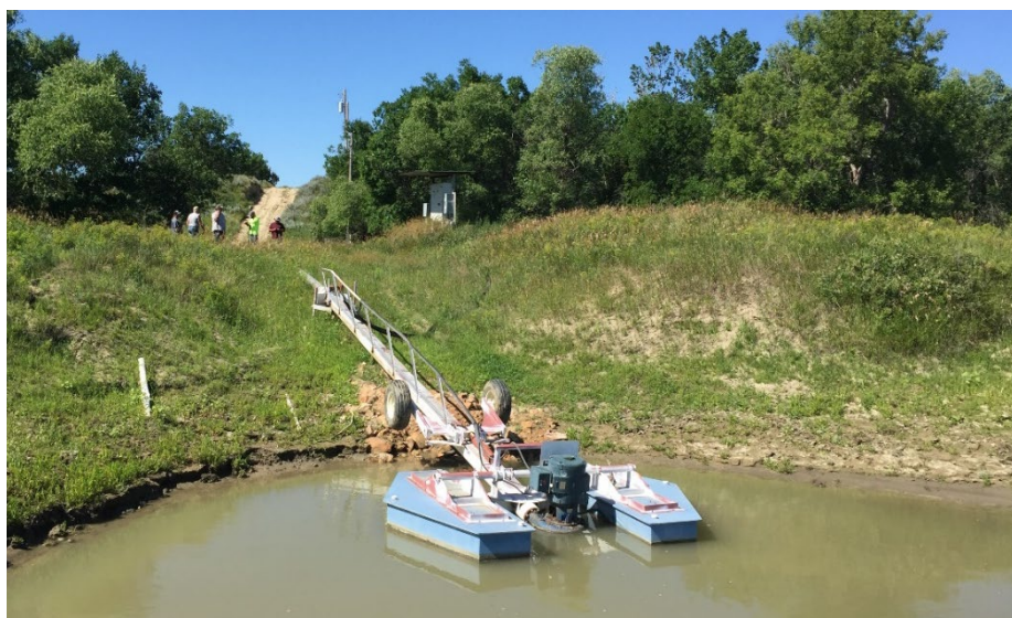
Figure 3-16. Typical pump intake located near RM 1760
