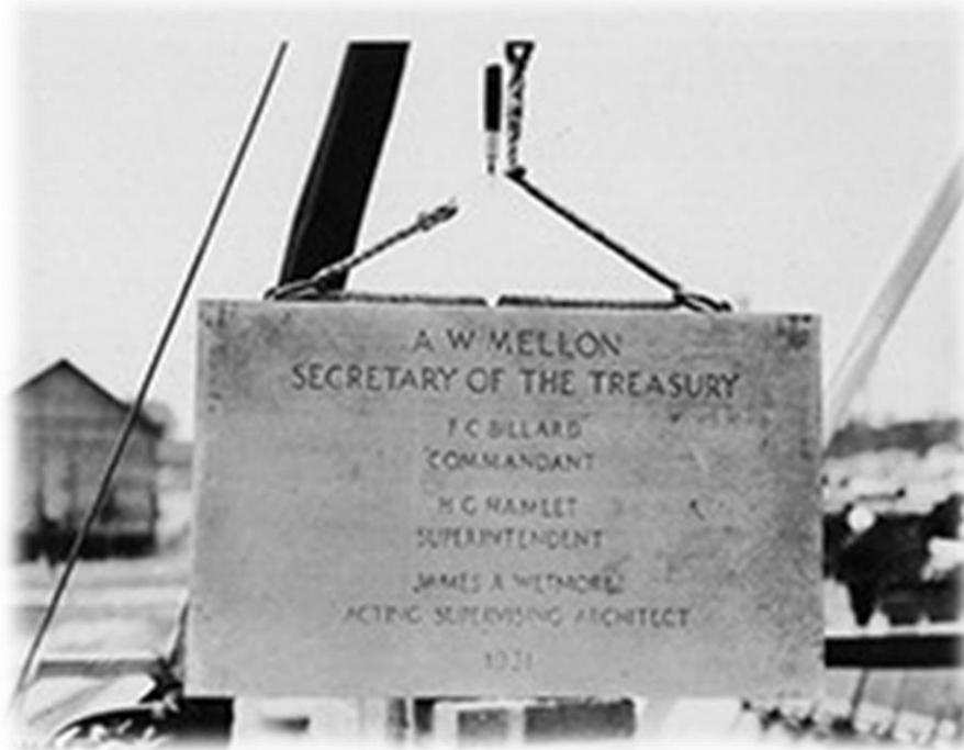
Laying of cornerstone for Hamilton Hall, United States Coast Guard Academy (CG photo)
