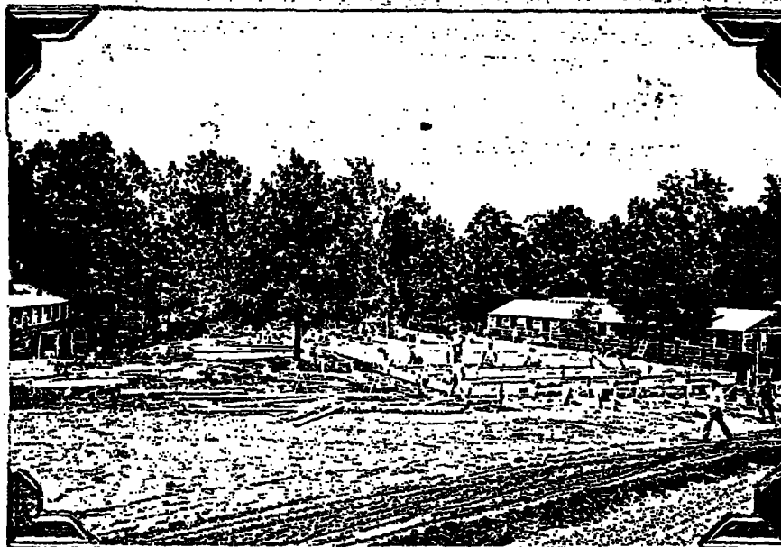
Construction of EM Barracks.
