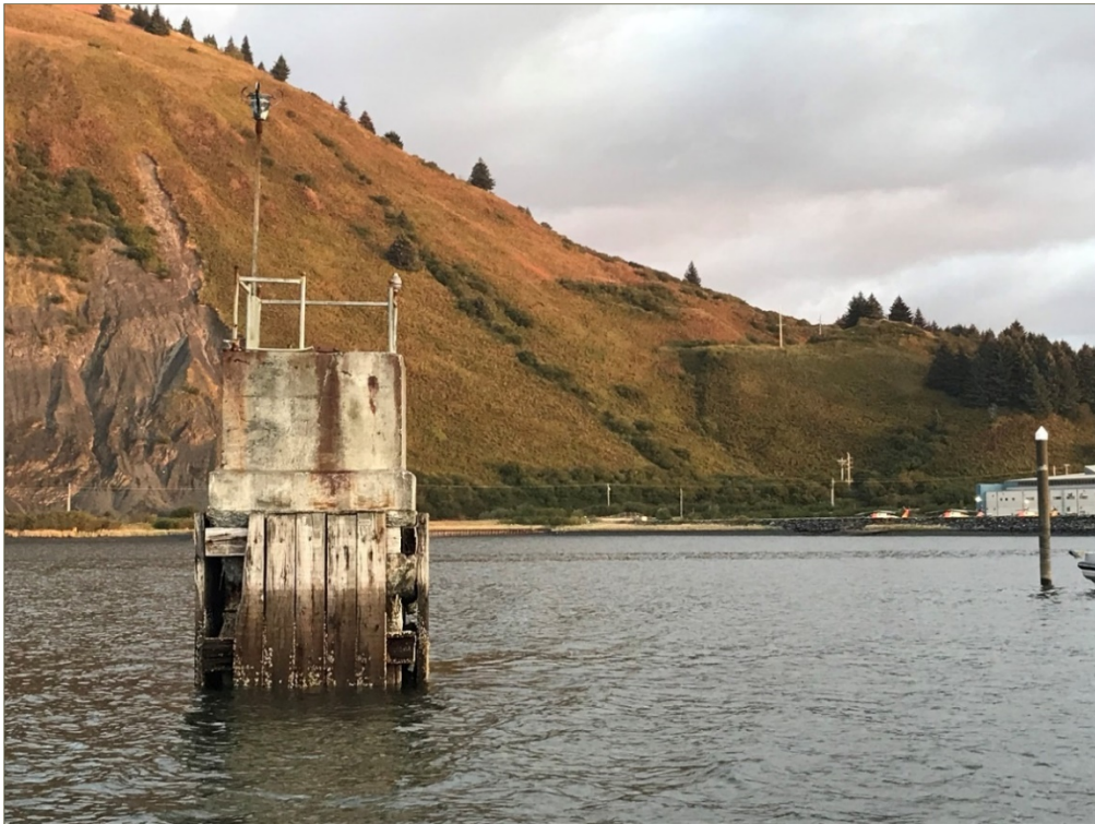
Exhibit 2.2-4: Photos of the Seawater Intake Structures on July 18, 2019 (Upper: Concrete Pile Cap in the Foreground and Intake Structure in the Background; Lower: Close-Up of the Intake Structure)
