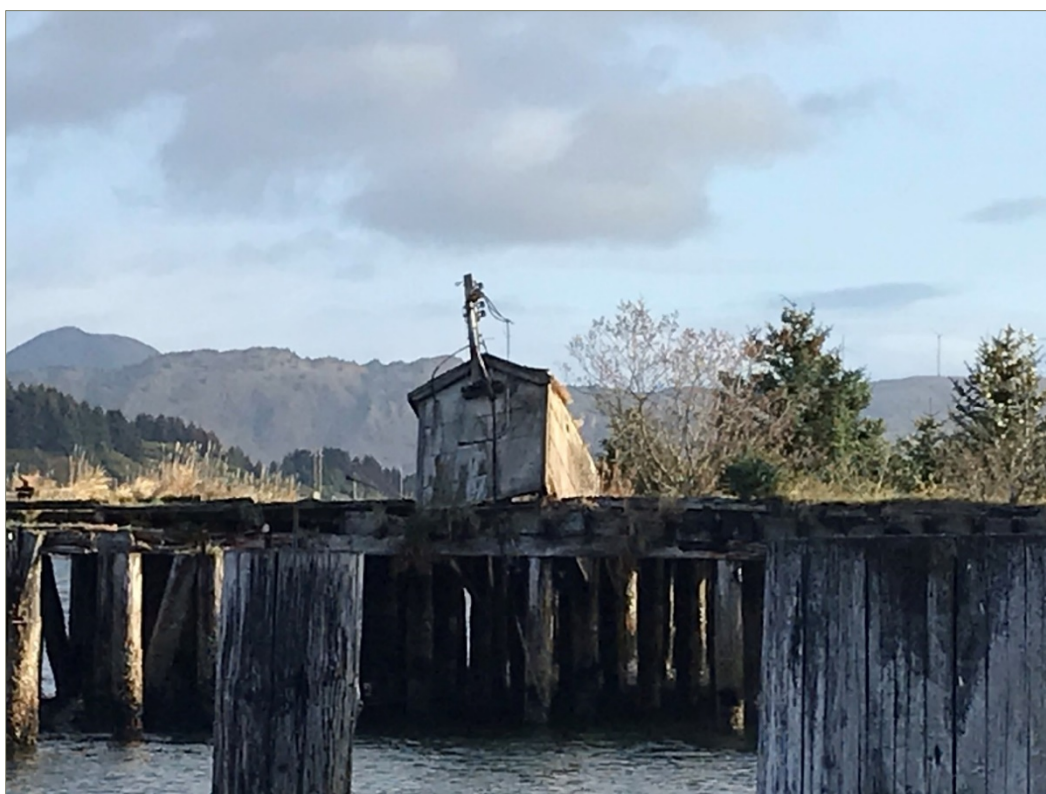
Exhibit 2.2-2: Photos of Marginal Wharf on July 18, 2019 (Upper: Old Conduit and Utility Structures; Lower: Shed with Cement Asbestos Board Siding)
