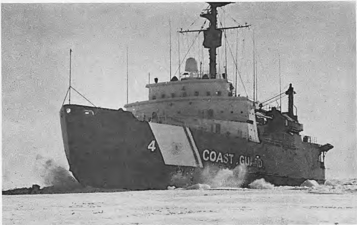
Plate 2. Channel break in, 3/4 ship length per ram in 6'-7' fast ice.
